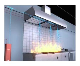
The Restaurant fire suppression system is a pre-engineered, wet-chemical, cartridge-operated, regulated pressure type with a fixed nozzle agent distribution network. It is listed with Underwriters Laboratories, INC (UL/ULC).
